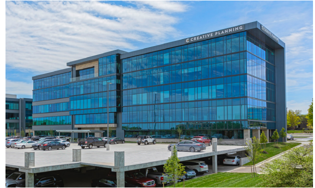
Overland One - Building 1
