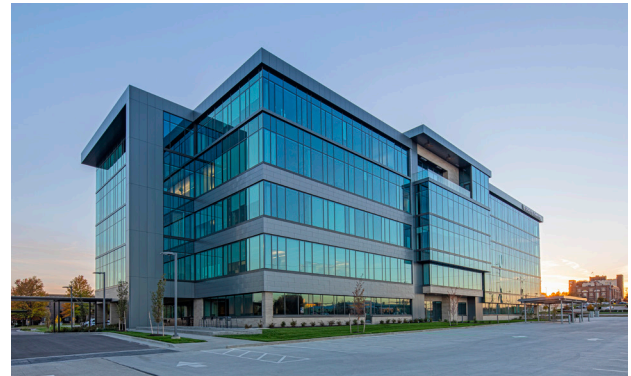
Overland One - Building 2
